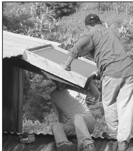
Patrick Delaney, helping to install a solar panel.
